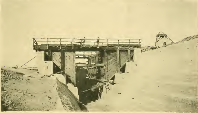
THE NEW ORE-BINS NEAR RIBBLESDALE SHAFT, MYSORE MINE.
