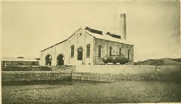
THE NEW COMPRESSOR-HOUSE, MYSORE MINE.
